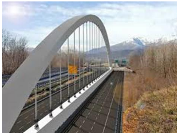
Figure 1. View of the suspended arch steel viaduct
