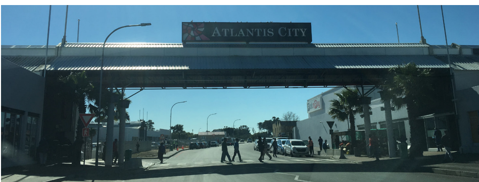
Figure 6.18 Atlantis commercial precinct centre 2019, Source; Author
