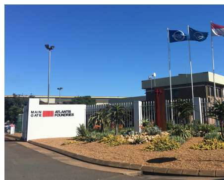
Figure 6.15 Atlantis industrial precinct 2019 , Source; Author
