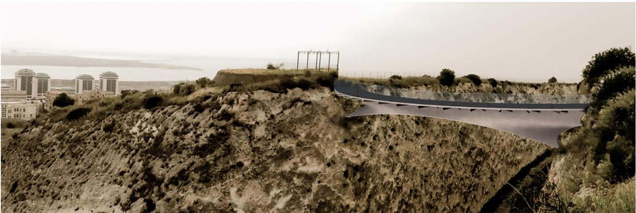
Figure 15: Photomontage of the curved shell-supported footbridge over Tuvixeddu canyon in Cagliari, Italy
