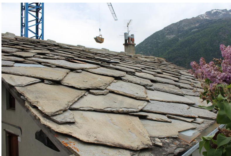
Figure 7. Calcschist CM roofing in Lignod after renovation.
