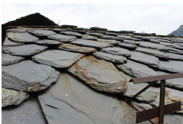
Figure 9. Old stone roofing in Porfiroide in Magneaz hamlet.
