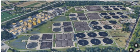
Figure 1: Photo of the WWTP.
