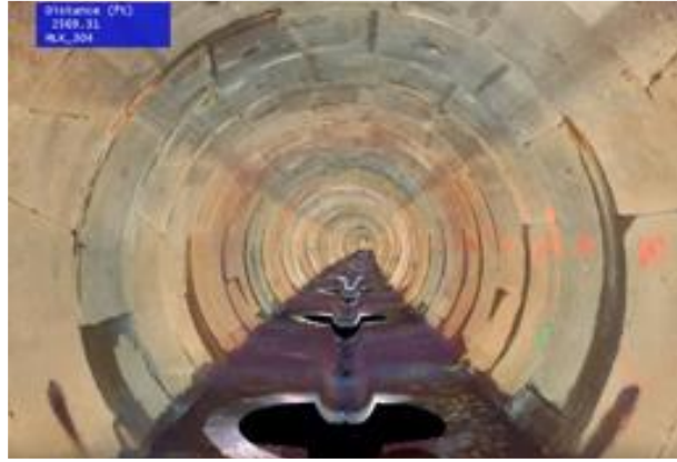
Figure 7. Color/Filtered Point Cloud of Tunnel
