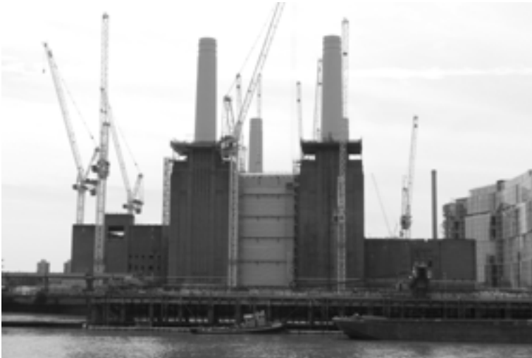
Nowadays. The construction site
