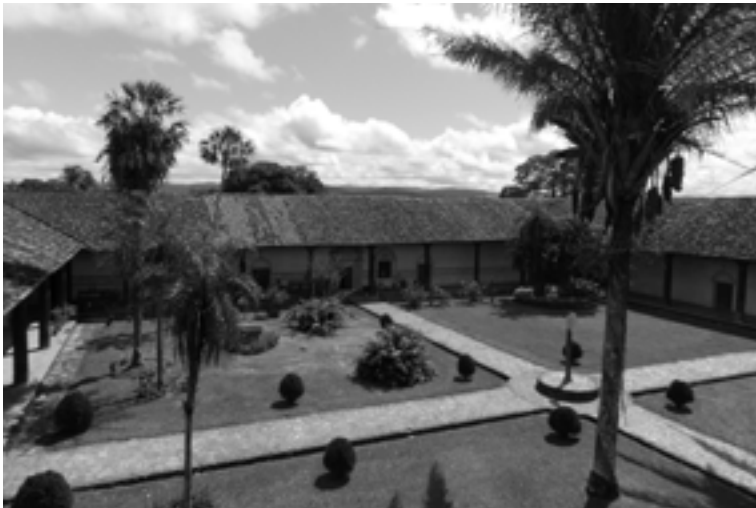
Surroundings of Concepción: traces of the past village.
