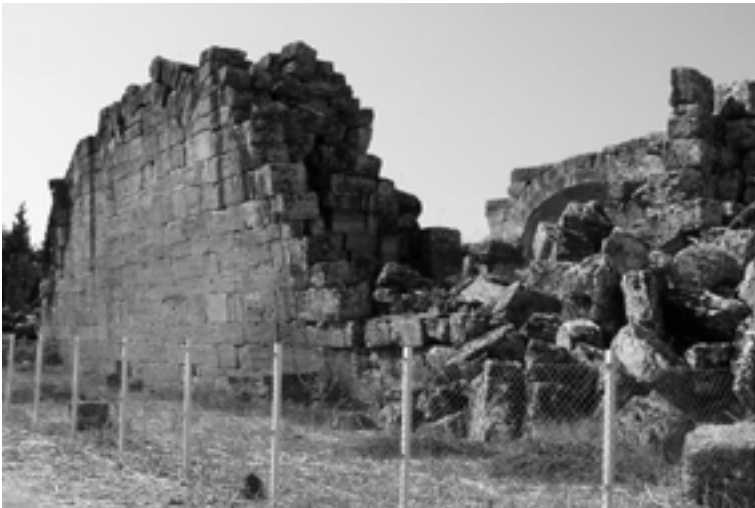
Hierapolis: the Thermae pillars deformed by the earthquake and the walls of the Thermae-Church deformation
