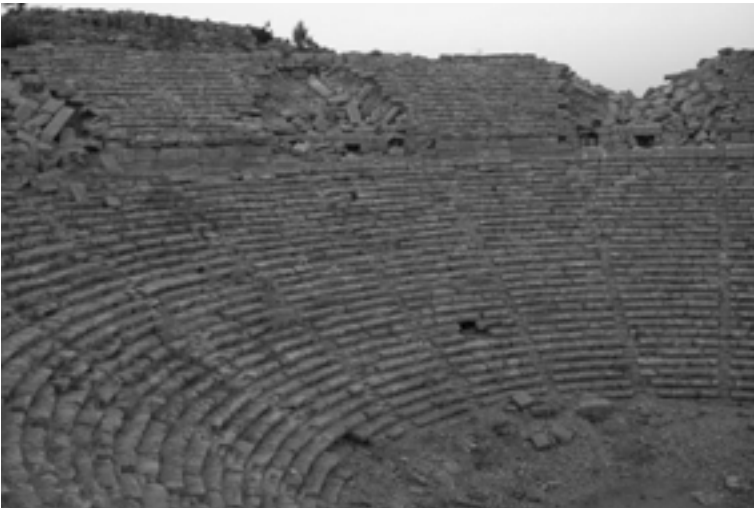
Didima and Selge: collapsed columns of the Apollo Temple and primary collapse in correspondence of the theatre cavea
