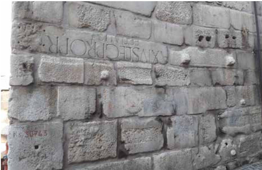
Reuse of roman parts in the Medieval structures.
