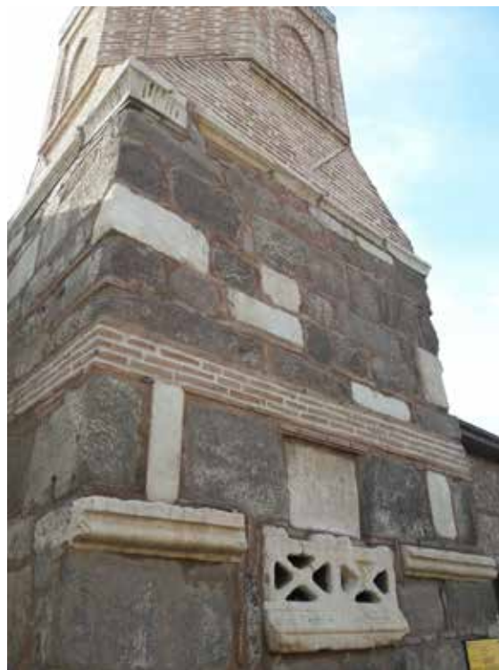
Roman ancient parts inside the construction of the minaret of the recent mosque near the citadel area.
