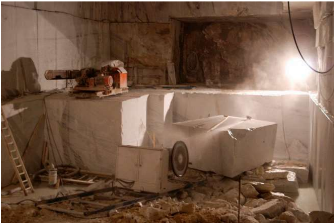
Figure 8. Chain cutting machine (on the top of the bench) operates in an underground extraction site (Lasa quarry), while a diamond wire saw performs a squaring operation.
