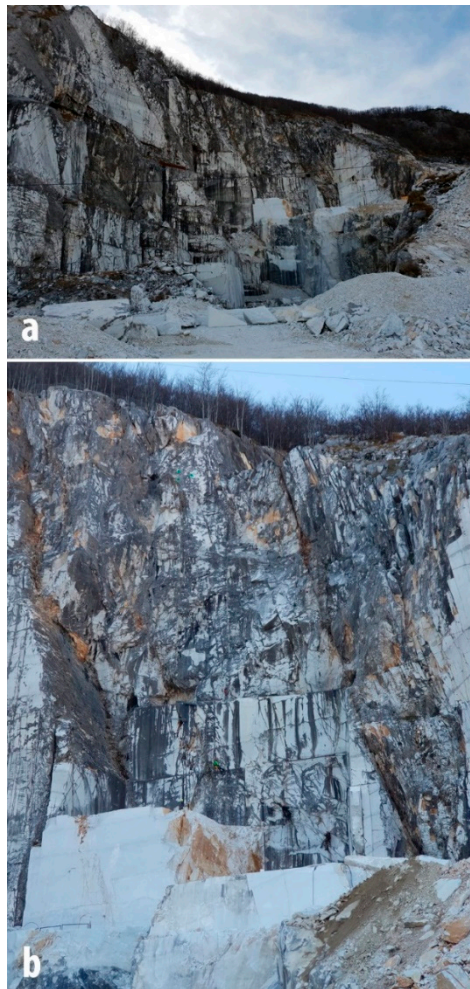
Figure 6. (a) strike-slip faults cross-cutting the Marmi s.s. Formation in the quarry area; (b) detail of the fault and damage zone.
