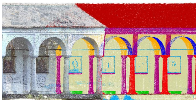
Figure 5. Example of moldings (purple) and columns (red).
