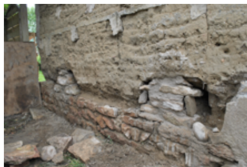
Fig. 2 - Raising the stone basement.
