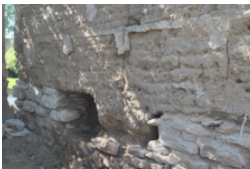
Fig. 1 - Hollowing out small portions of rammed earth wall.
