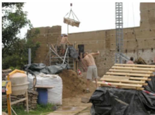
Fig. 7 - Soil pouter in action.
