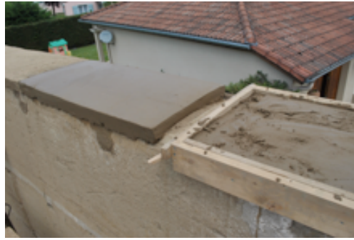
Fig. 5 -Slipping formwork.
