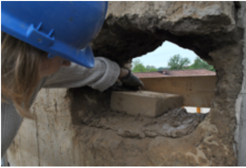
Fig. 4 -Filling in holes in rammed earth.
