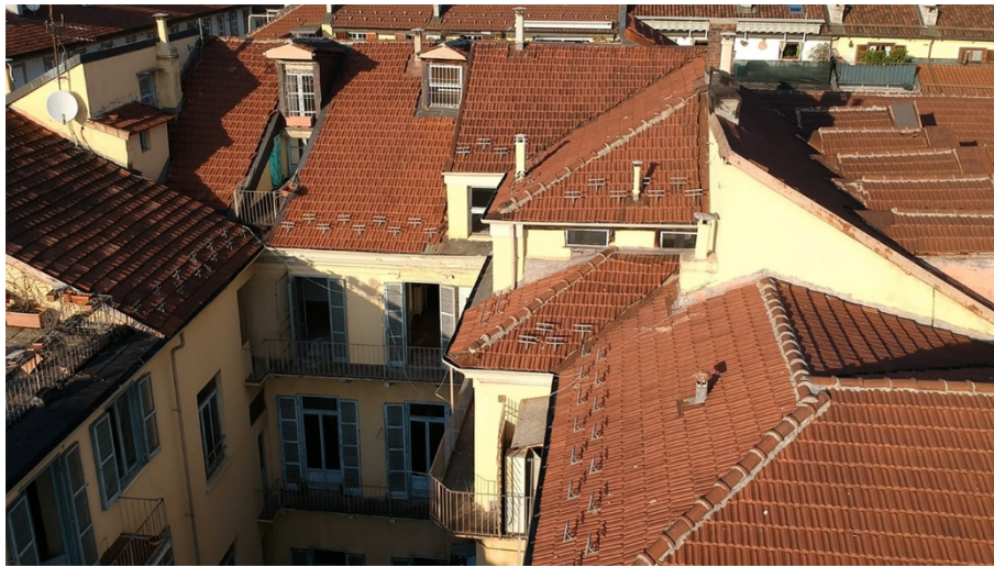
Figure 7. Picture that shows the facade of the inspected building. The frame was extrapolated from the video registered by the UAV's camera (source: real estate company archive).
