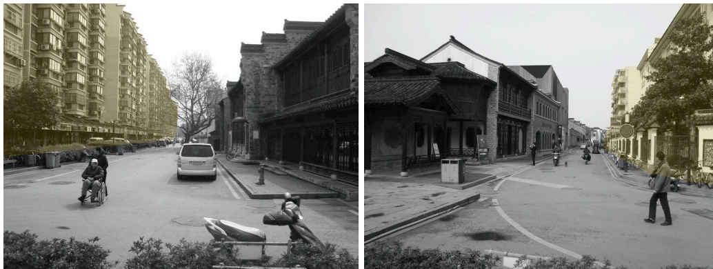
Figure 93 Buildings height along Jianzi Alley (by author)
