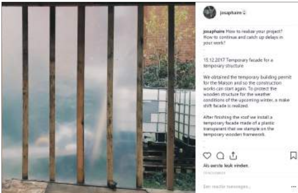
00.08.fig.16 - TL.15.12.2017 Temporary facade for a temporary structure.
