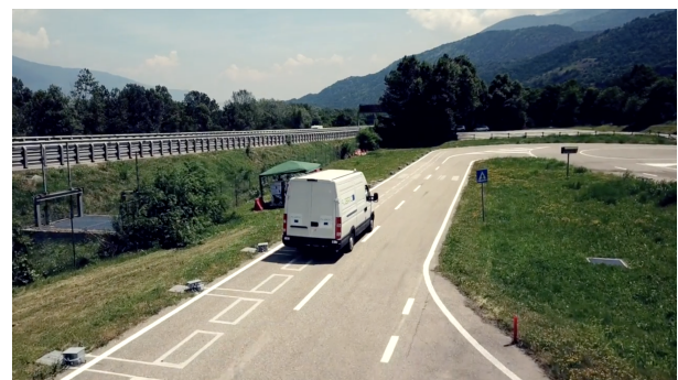
Fig. 16: The EV in the charging lane.
