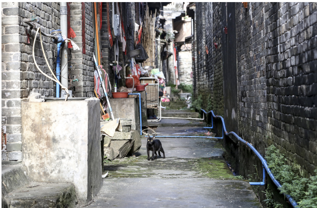
7.9 | External pipes in rural villages of Zhaoqing. Samuele Pellechia. 2017
