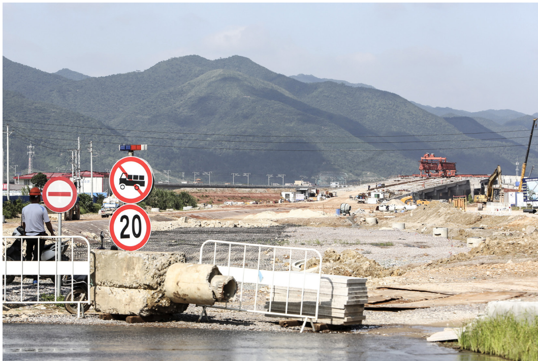
3.18 | Evolution of roads construction within Zhaoqing New Area. Samuele Pellecchia. 2017
