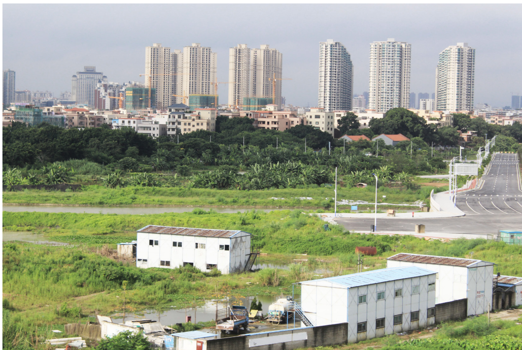
8.3 | New roads connecting the peripheries in Foshan. Photo by the author. 2018
