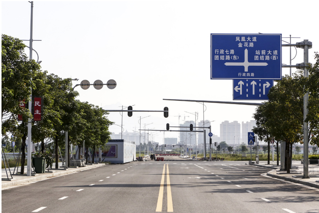
3.16 | Deserted roads within the construction site Zhaoqing New Area. Photo by the author. 2018
