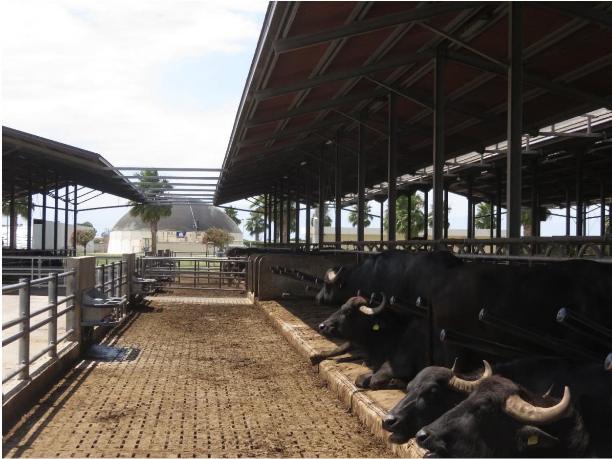
Figure 36. Biogas plant at a large, modern buffalo farm near Battipaglia, Province of Salerno (photograph by the author)
