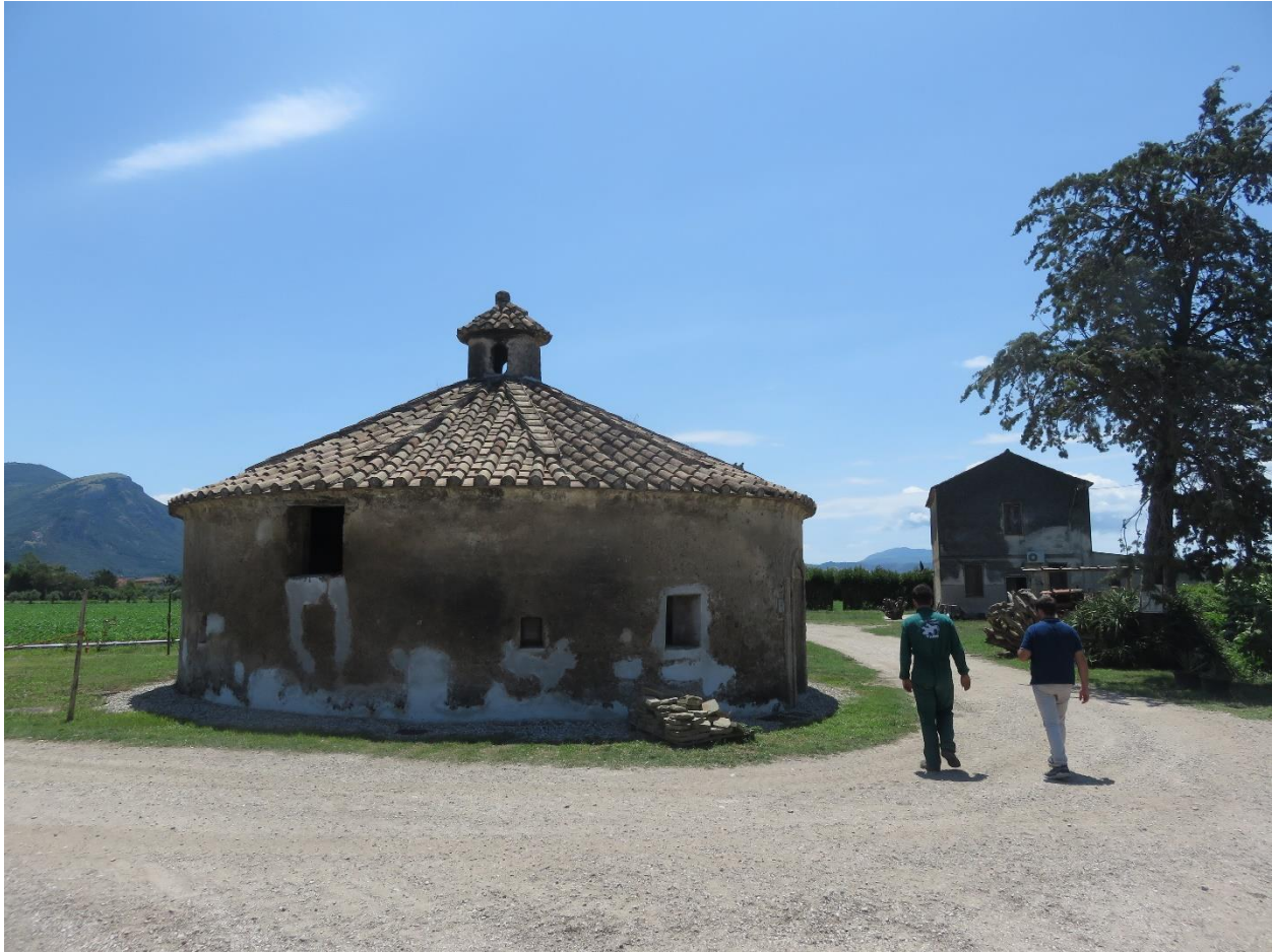
Figure 15. A 'bufalare' on a buffalo farm near Battipaglia, Province of Salerno. These characteristic circular shaped masonry constructions date back to the 15 th century. (photograph by the author)
