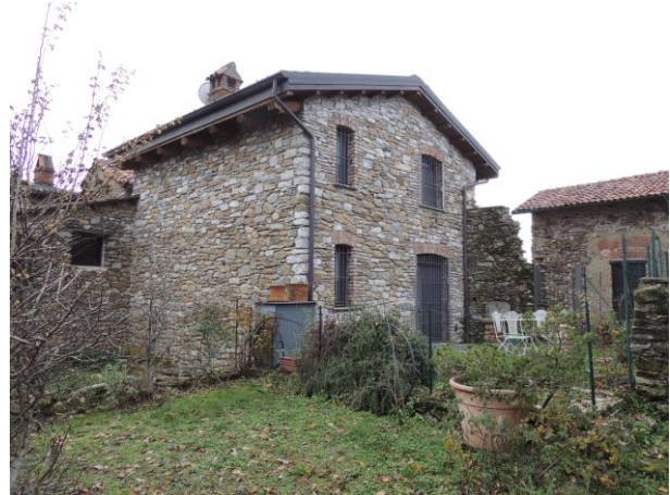
Figure 10. Building D - Reintegration of the upper part of the walls and of the roof (credits Manuela Mattone).
