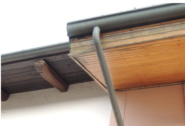
Figure 9. Building E - Wooden battens in the overhang of the roof (credits Fabio Fratini).
