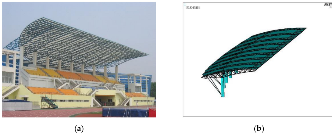
Figure 9. Stadium stand hood model: (a) Real image; (b) finite element model.
