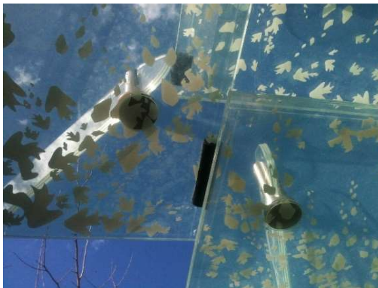
Figure 1: Example of building with glass and steel: particular of the glass panel with the adhesive joint glass/steel.
