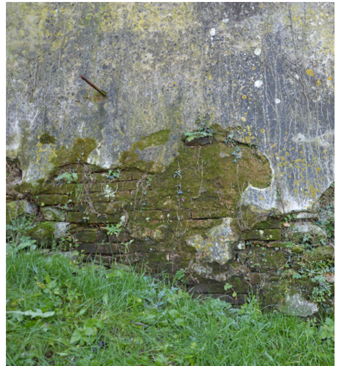
Fig. 2. Serralunga di Crea, Sacro Monte, Chapel 1. Main façade (right) and damage at the base of the northern façade (left).
