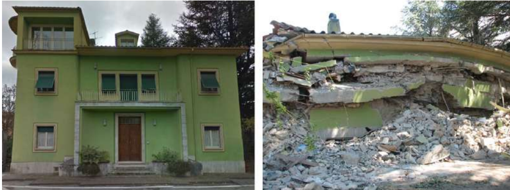
344 345 Figure 10. View of the building used as case study before and after the earthquake.
