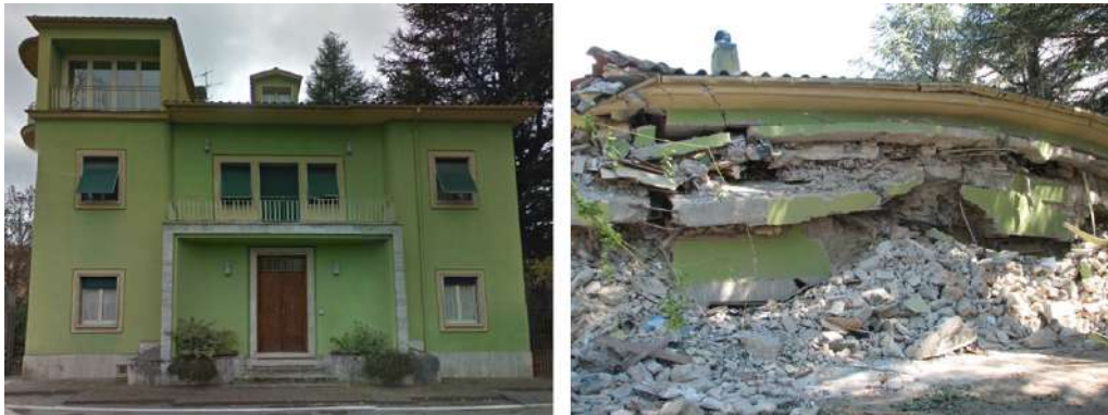
787 345 Figure 10. View of the building used as case study before and after the earthquake. 788 789 346
