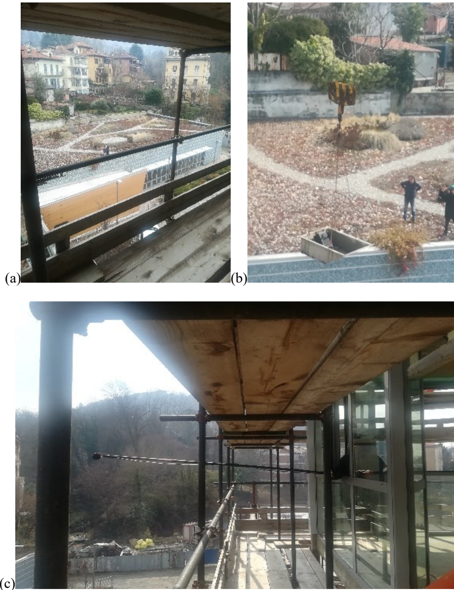
Figure 6.19- (a) first attempt of positioning of the sound source, as seen from inside the indoor environment; (b) repositioning the sound source with the crane; (c) positioning of the outdoor receiver.
