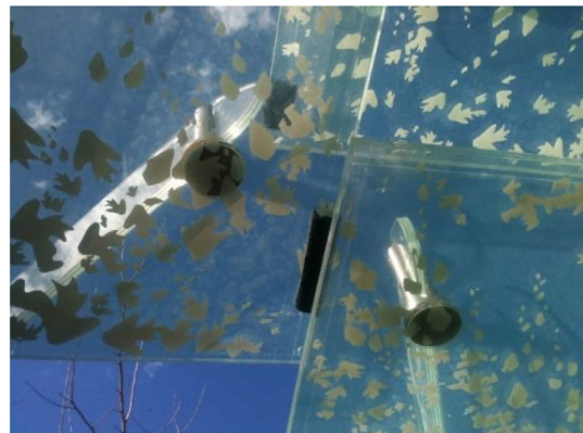
Fig. 1. Example of building with glass and steel: particular of the glass panel with the adhesive joint glass/steel.
