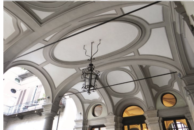
Figure 4. Banded vault with independent arches in Palazzo Barolo (top) and with arches belonging to the main surface in the palace in via Garibaldi 53 (bottom). Photos: M. Vitali
