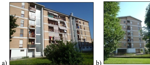
Figure 2: Building façades. a) East; b) North.
