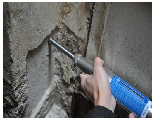
Figure 6. Constructional element identification using concrete hammer test
