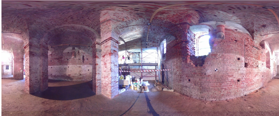
Figure 73. Panoramic image from laser scanner (2018 survey): inside the refectory
