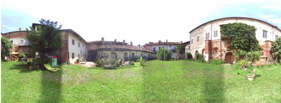
Figure 75. Panoramic image from laser scanner (2018 survey): south front of the refectory
