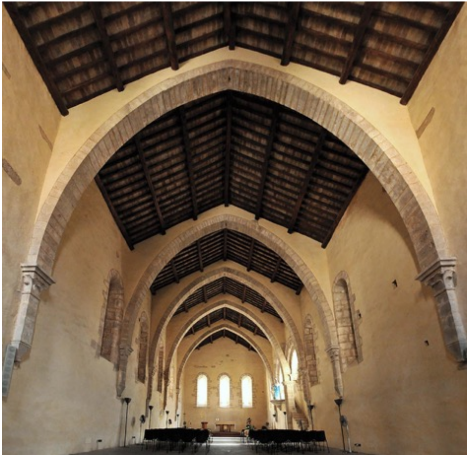
Figure 28. Fossanova refectory and its ceiling (From E. Gallotta, 2018, photo A. Grella)
