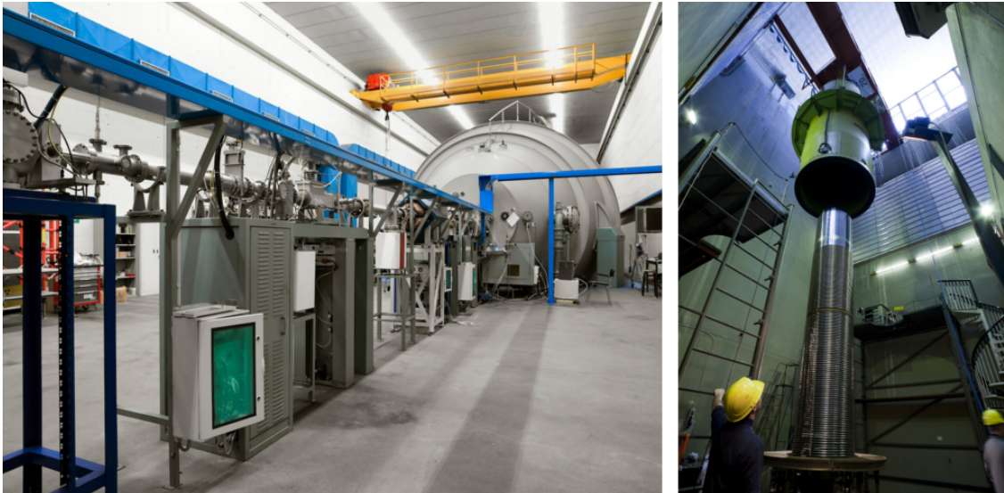
Figure 3.3: Pictures of the Tandem XTU accelerator and outgoing beam pipe on the left and of the tower of the CN accelerator on the right. Courtesy of Andrea Alessio.
