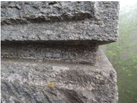
Fig. 8. The angular ashlars (Fratini).
