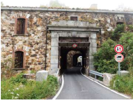
Fig. 4. The access to the tunnel (Fratini).
