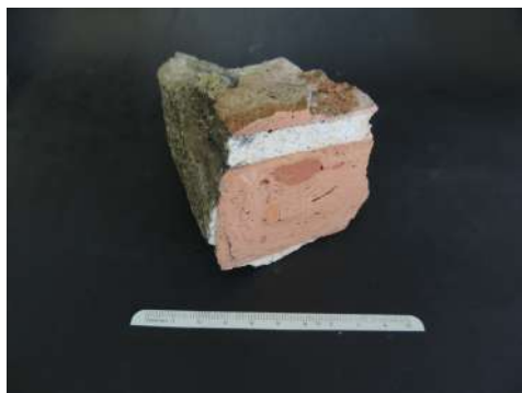
Fig. 17. Bricks of the frame of the openings (Fratini).
