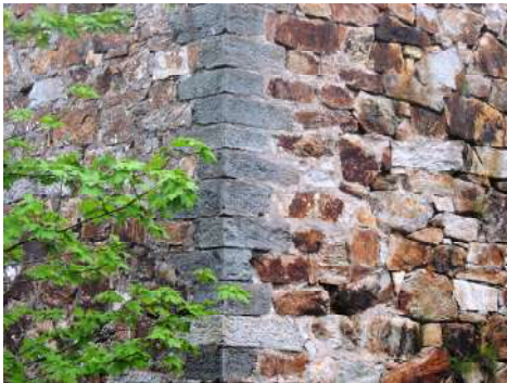
Fig. 5. The corner headboards (Mattone).
