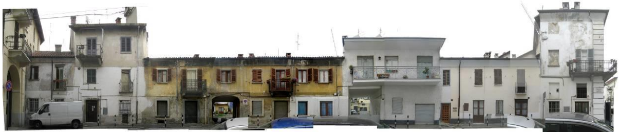
Fig. 8: Photogrammetric straightening of the façade overlooking via Cesare Battisti.
