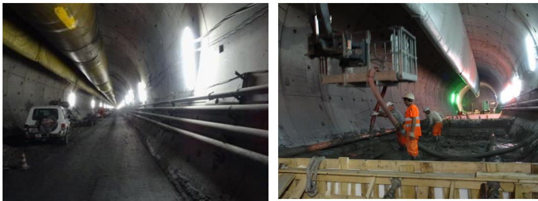
Figure 5.7 New tunnel under construction at Frejus
