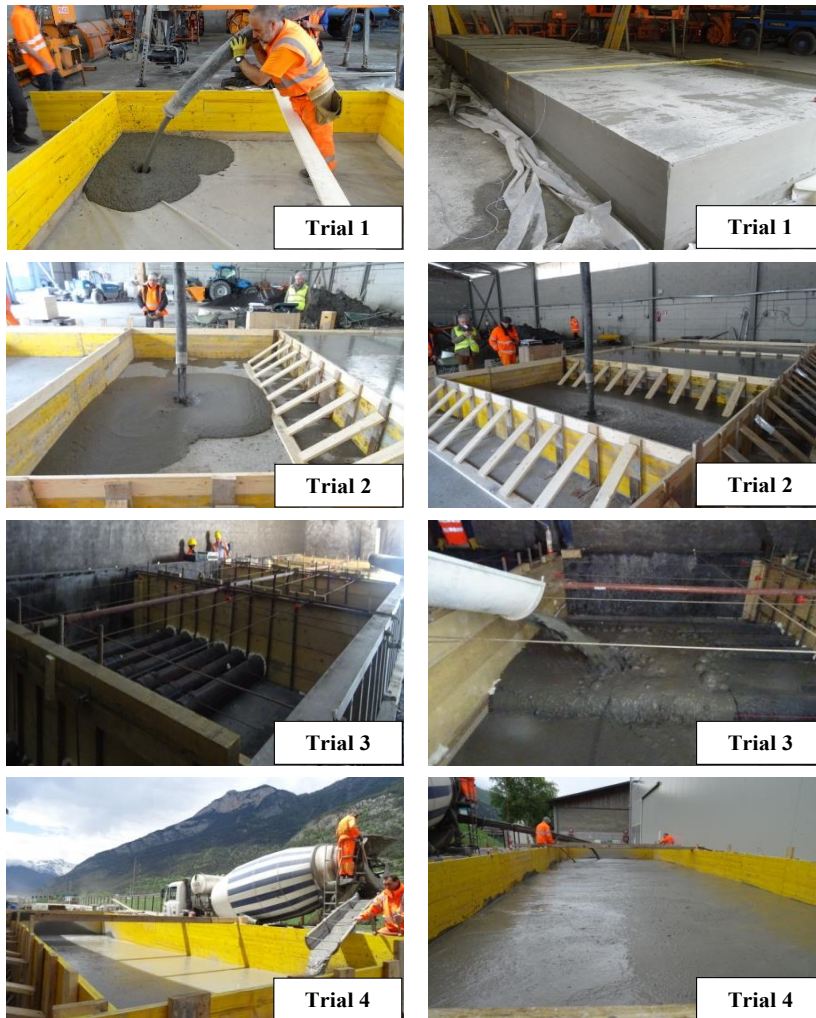
Figure 4.7 Construction of slabs in field trials.
