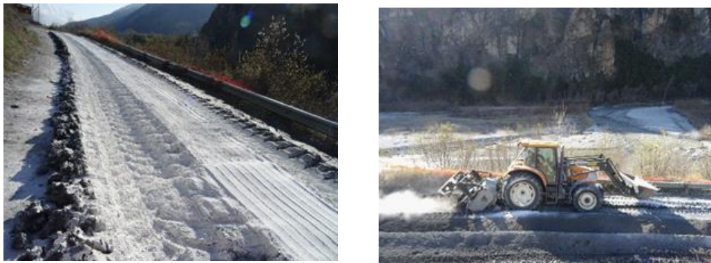
Figure 4.2 Sludge drying at the field using pulvimixer
