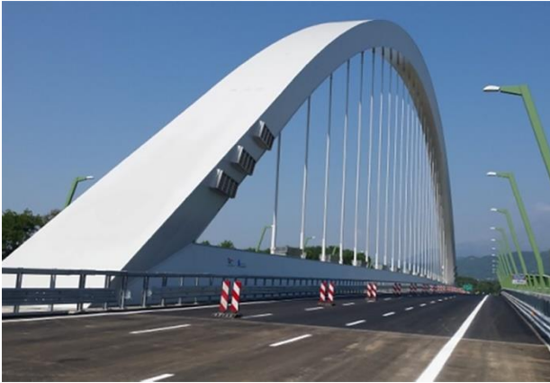
Fig.1 General view of the bridge
