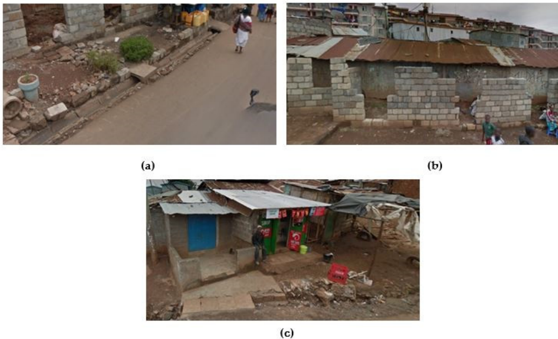
Figure 20. Hot-spot 2: territoriality elements. Drainage system (a), abandoned building structure (b), and porticos (c) (source: Google maps street views).
