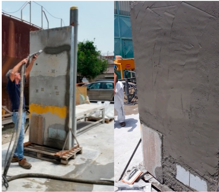
Figure 5. Left: Plaster pouring on a vertical panel. Right: results after pouring.
