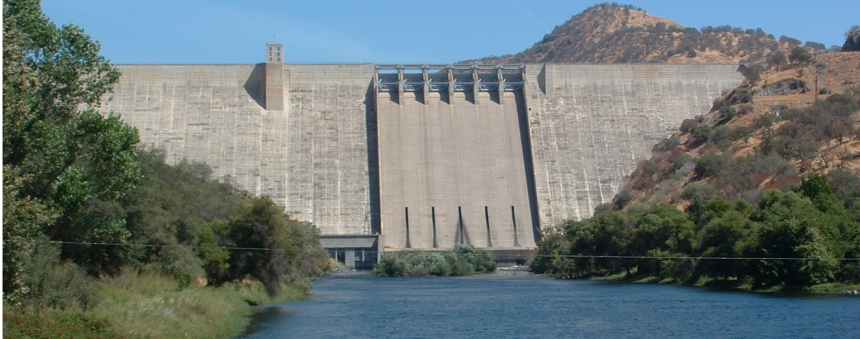
Figure 1 Downstream view of Pine Flat Dam [ref. Wikipedia.org]
