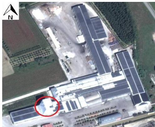
Fig. 2. Satellite image of the 2.5 MWp BIPV system.
