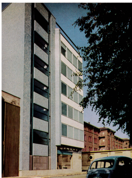
Figure 1. Domenico Morelli, SIP Office Building, Turin, 1951-57 (with T. Finzi; structure by A. Antoldi; construction company: Rain-eri). The face of the prism overlooking Via Promis is distinguished by the vertical stair block [2].
