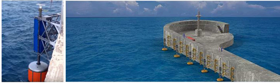
FIGURE 10 | WEC module (Left) and schematic representation of port of Heraklion, Greece (Right) © SINN Power.
