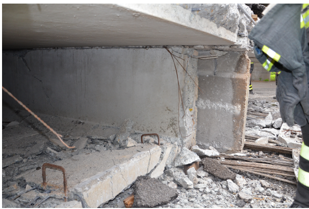
Figure 2: Collapsed joint.
