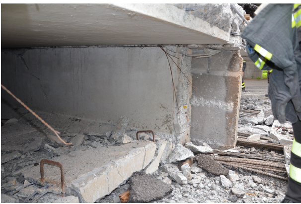
Figure 2: Collapsed joint.
