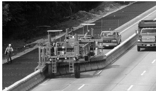
Figure 29 - mechanized “Barrier Zipper” technique.
