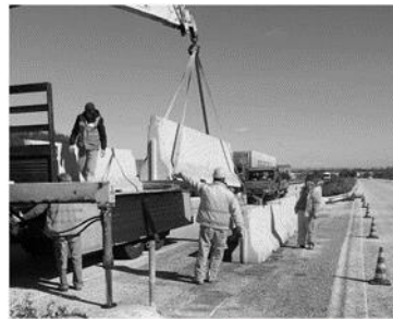
Figure 28 – barrier transfer: traditional procedure
