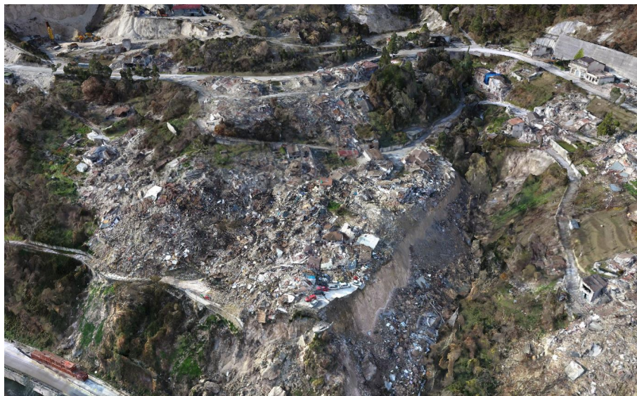
Figure 6. Model of Pescara del Tronto after the October 2016 Earthquake events.
