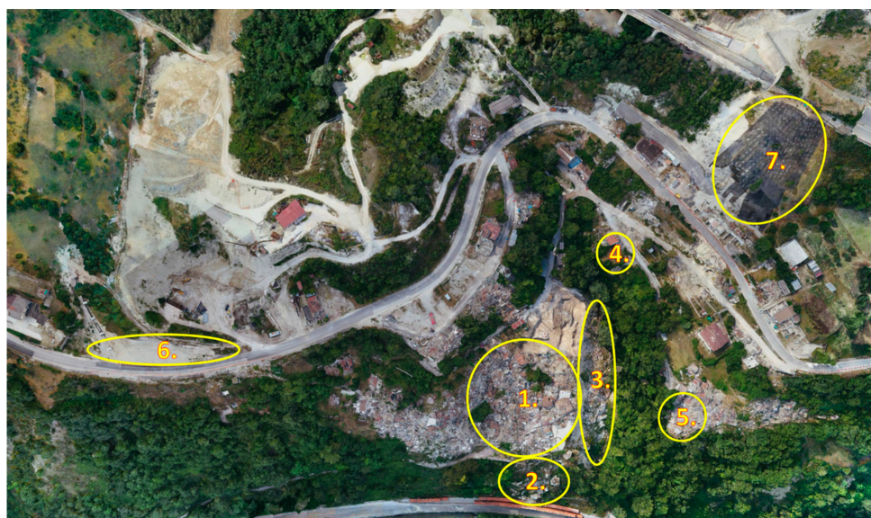
Figure 16. Pescara del Tronto Locality Map (similar to GEER map) [1]. Areas of Focus: 1—Structural Damage of Residential Area, 2—Landslides Impacting the Strada Statale, 3—Failed Retaining Wall Surrounding the Village, 4—Localized Landslides along the gully wall, 5—Landslide on Northern Slope of the Village, 6—Haul Road and Exposed Pipeline, 7—Large Slope Failure North of the Village.
