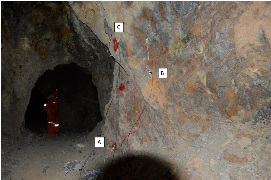
Figure 4. Installation of the sensors on the tunnel walls. Each sensor lay on a joint belonging to a different set of discontinuities.
