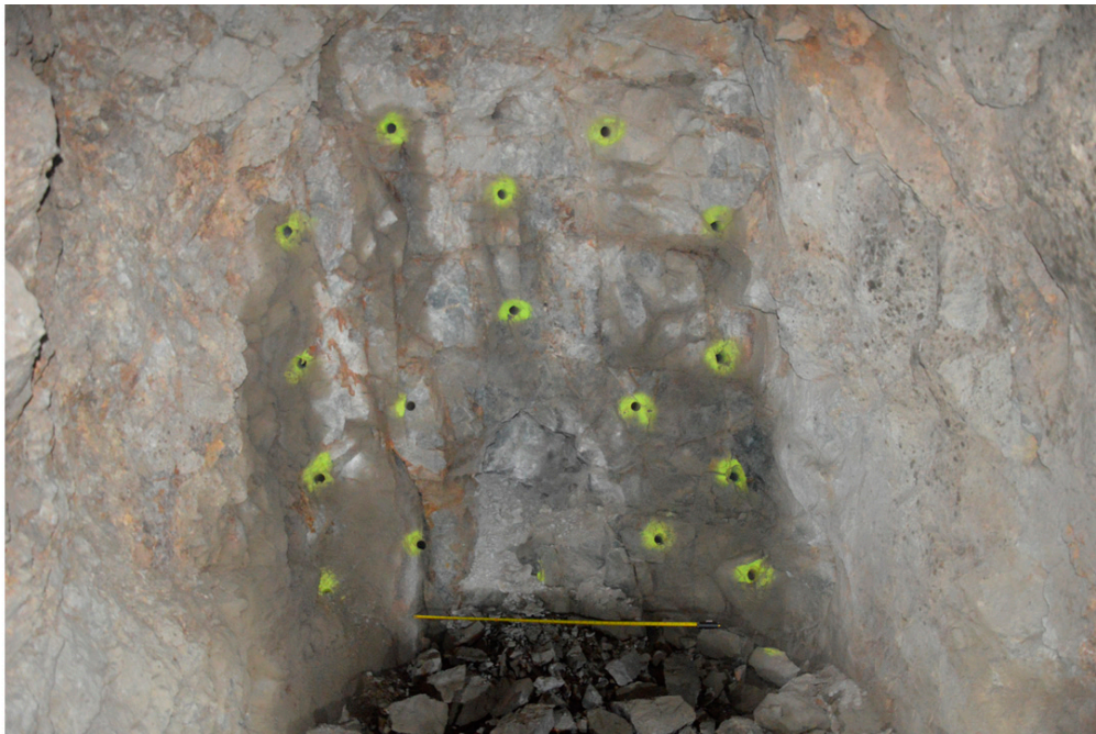
Figure A5. Cavity after detonation of hole with sequence number 4.
