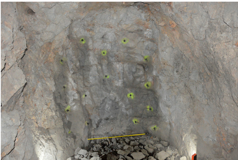
Figure A6. Cavity after detonation of hole with sequence number 5.
