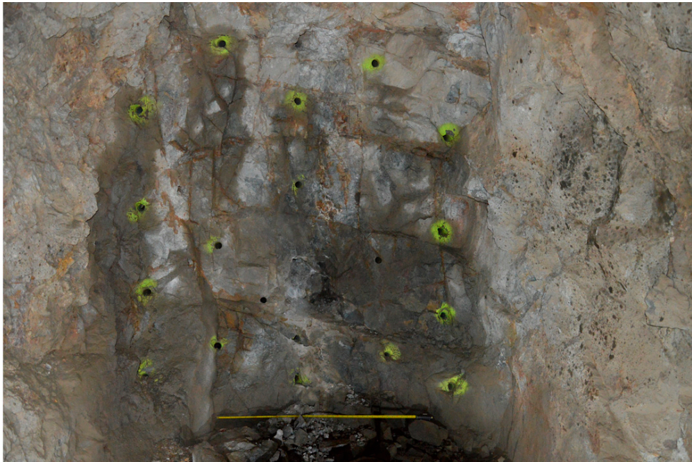
Figure A3. Cavity after detonation of hole with sequence number 2.
