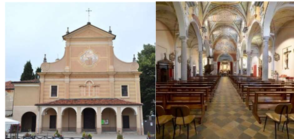
Figure 2a and b. Facade and naves of the Church.
