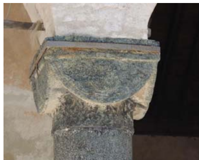
Fig. 03 : Serpentinite in regular blocks (on the left) and in column and capital (on the right)
