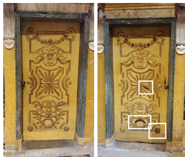
Figure 3a and b. The reference door used for the survey (left) and the ruined one (right) with the identification of the missing elements.
