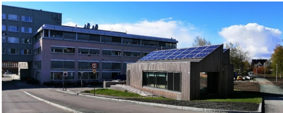
Figure 1. The ZEB Living Laboratory and its surrounding.
