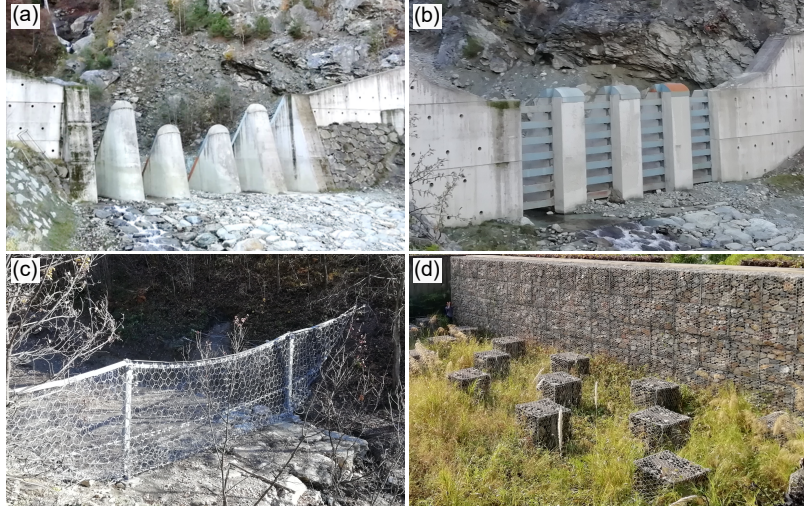
Figure 1: Examples of debris flow mitigation structures, with energy-breaking or filtering function. (a) Front breakers and (b) slit-filter barrier installed in Pollein, Aosta Valley, Italy. (c) Flexible steel-ring net installed in Bussoleno, Piedmont, Italy. (d) Debris-resisting baffles near Yu-Thung Road, Hong Kong, HKSAR.
