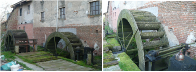
Figure 1. The existing breastshot water wheels, for which a 1 : 2 scale model was investigated in this work. The original diameter is 4 m.
